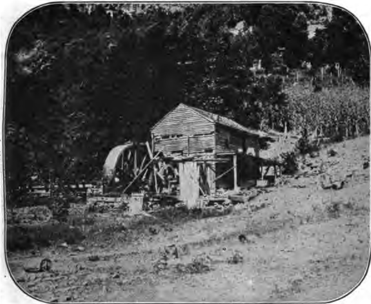
FIG. 101.—Abandoned grist mill in Tennessee. Old-fashioned overshot water-wheel, cornfield in background.
